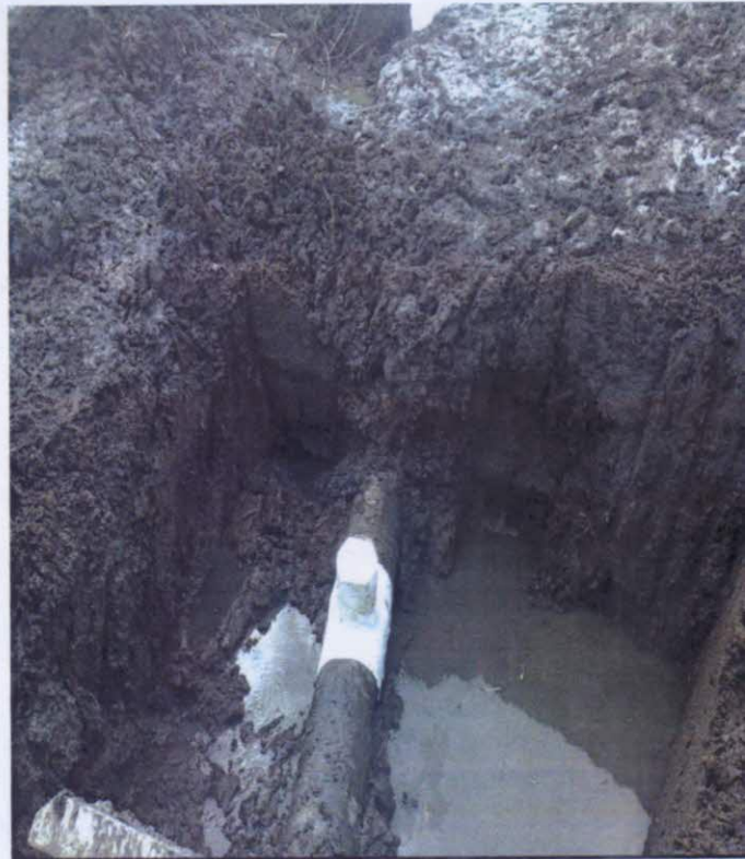
F.g 2. After Repairs
