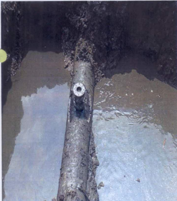
F.g 1. During Repairs
